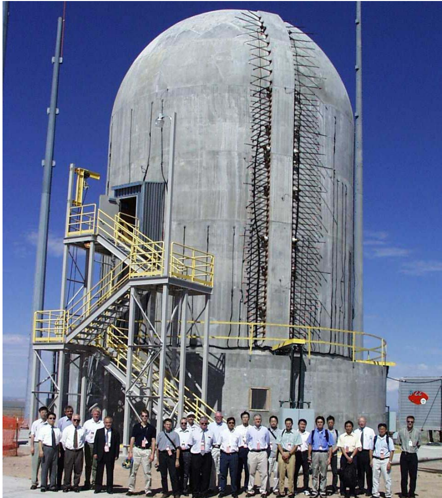
Figure 1.- Photograph of the PCCV
