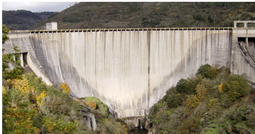
FIGURE 4: General view of the double curvature arch dam
