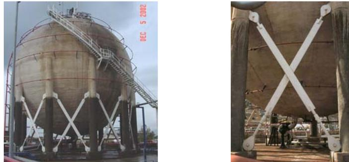
Figure 1 Selected sphere and detail of the tension-only bracing system.
